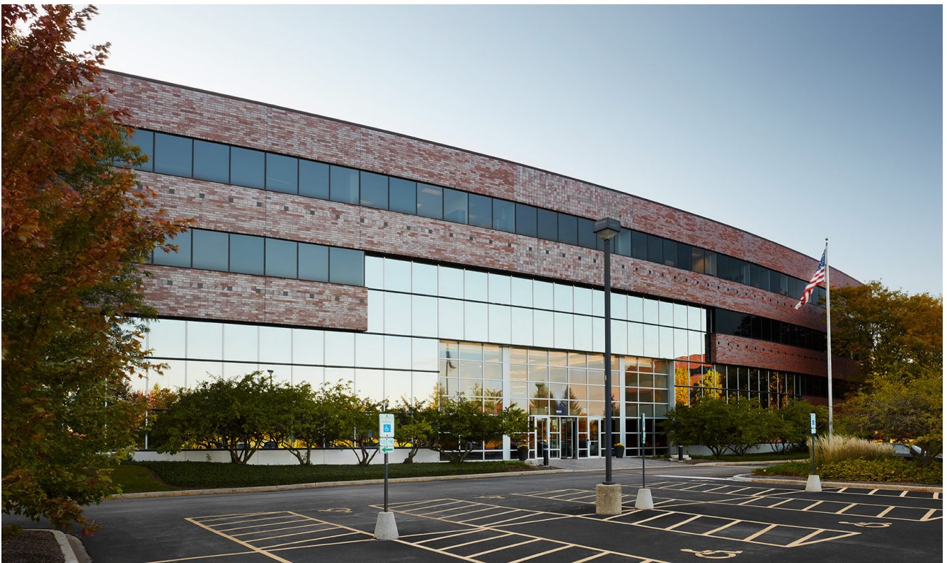
Kensington Corporate Center in Mount Prospect, IL, an Office & Medical Office Building for which JDJ Architects is providing Landlord Architect Services
